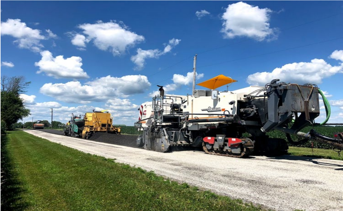
Figure 23 CIR Mix Being Delivered to Paver via Windrow (Courtesy HRG)
