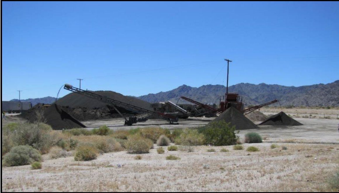
Figure 6 Fractionating RAP (Courtesy ARRA)
