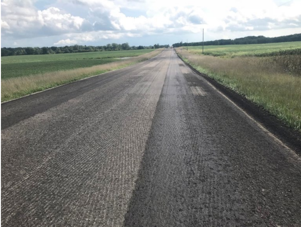
Figure 26 CCPR After Scarification Milling (Courtesy HRG)
