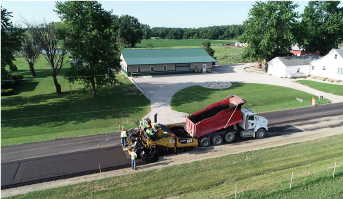
Figure 23 CCPR Mix Being Directly Delivered to Paver (Courtesy HRG)
