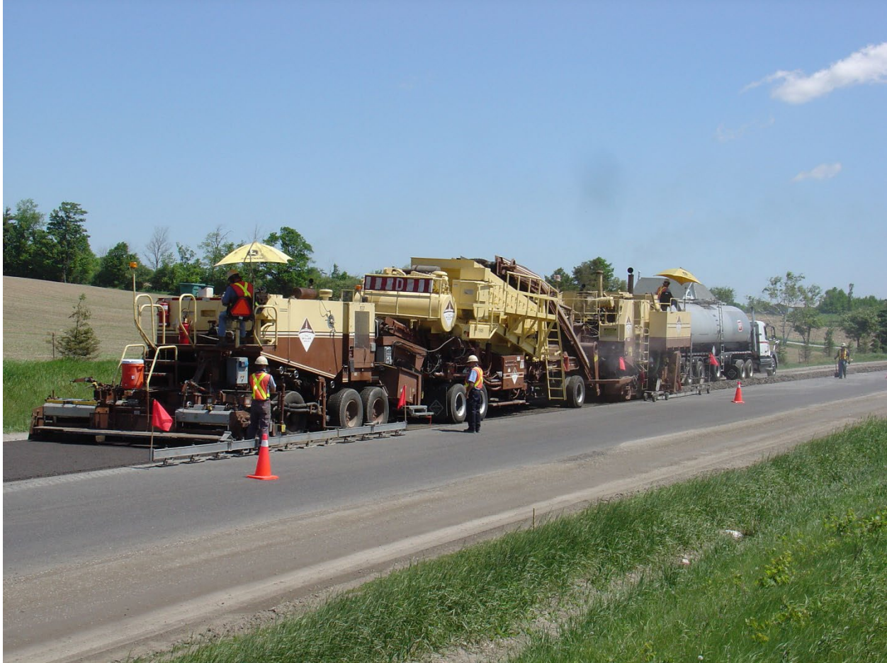
Figure 16 Multi-unit train (courtesy ARRA)
