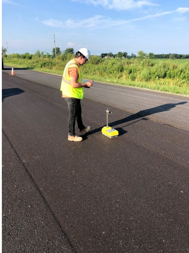
Figure 27 Nuclear Density Testing (Courtesy HRG)
