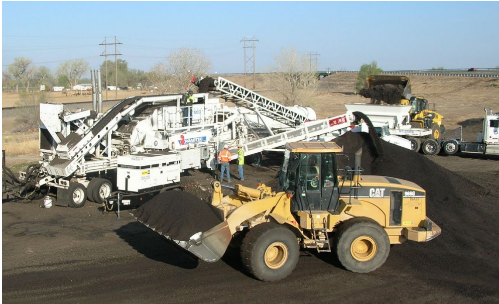
Figure 19 Processing unit from multi-unit train producing CCPR mix (ARRA 2015)
