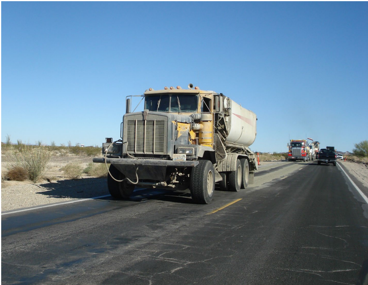
Figure 11 Applying active filler (cement) ahead of a multi-unit CIR train. (courtesy ARRA)
