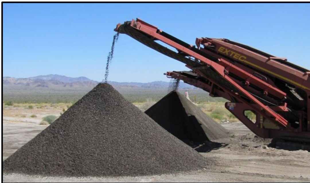
Figure 5 Fractionating RAP (Courtesy ARRA)
