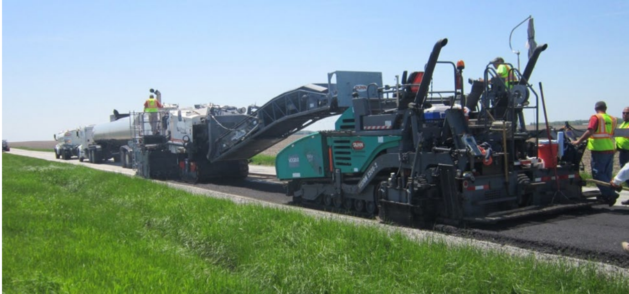
Figure 13 Single Unit CIR Train (courtesy HRG)
